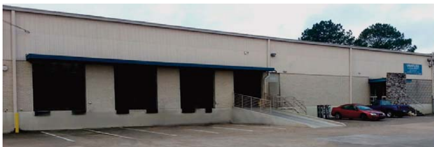
Houston, TX Warehouse Facility
